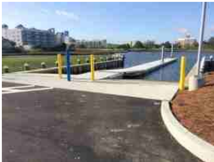
Funding for public ramps should be a big priority as it increases water access to the general public and can be used by car-top boaters. (photo: Maryland DNR)
